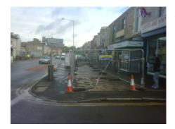
A culvert partially collapsed, holding back water which over-topped river walls and flooded property in the Blackburn Road and Duckworth Street. Urgent repair works are ongoing at a cost of £460k. The Clarence Street culvert, which carries the River Darwen, experienced a blockage and partial collapse. This to be 240 metres downstream of the culvert entrance where service pipes run across it - the culvert is over 500 metres long and working conditions are difficult.
